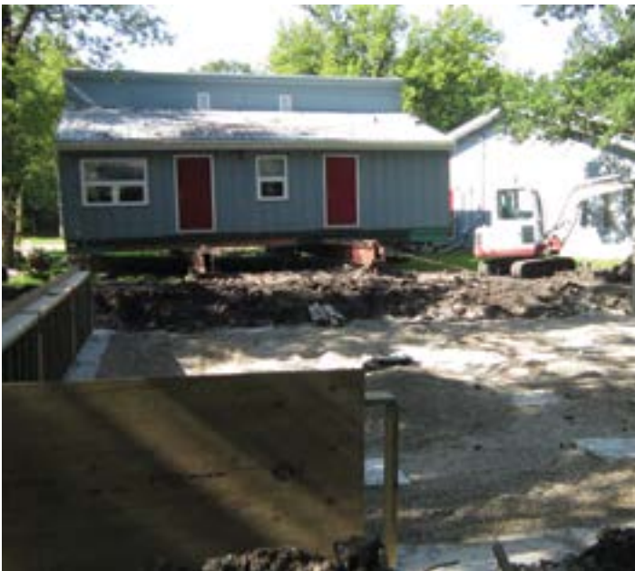
Replacing the foundation under Lodge 1 was a big job!
